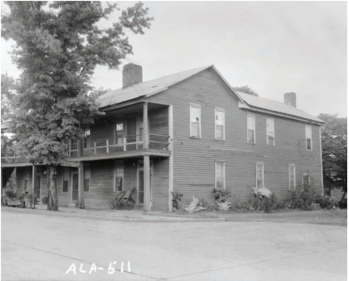
The United States Hotel, run by the Dennis family, circa 1935, looking much as it would have during the antebellum period. (W. N. Manning, Historic American Buildings Survey / Wikimedia Commons)
